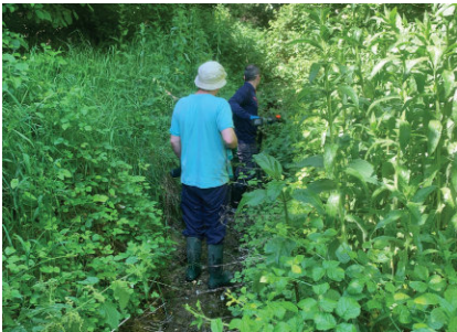
Clearing out Fox Brook to ensure the rainwater flows smoothly
