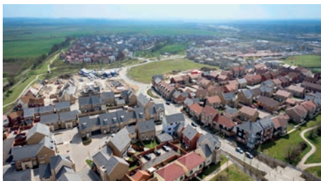
Love's Farm under construction, back in 2013
