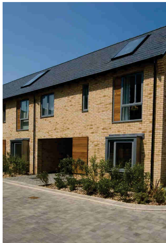
Consistent angle of roof pitch along a terrace
